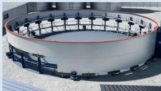
4. Feed in and tack weld the 2nd course, lower Jack one by one during the infeeding of the sheet.
