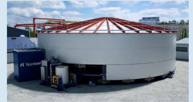
6. Assemble the 3rd course and so on until the tank reaches the final height. All NDT can be performed at ground level from one location. Remove the equipment, lower the tank to the bottom and dismantle the Lift Jacks.
