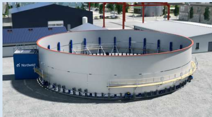
4. Assemble the 1st course including the top ring. Lift the 1st course, assemble and weld the 2nd course.
