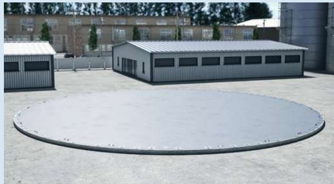
2. Place the annular and bottom plates at the foundation.
