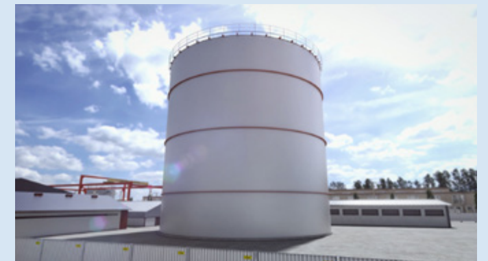
10. The tank is ready to use.
