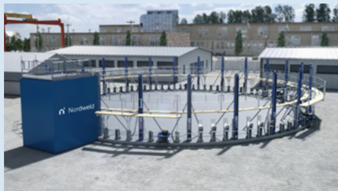
3. Place the equipment at the annular plates and assemble the Lift Jacks.
