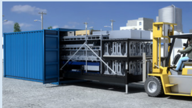
1. Unload the container.
