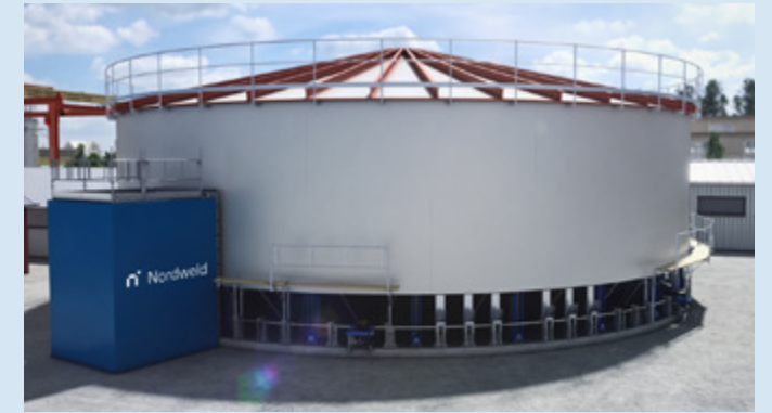
6. Lift the entire tank.
