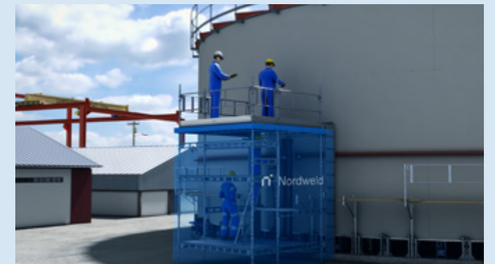
8. All NDT can be performed at ground level from one location.
