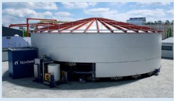
6. Assemble the 3rd course and so on until the tank reaches the final height. All NDT can be performed at ground level from one location. Remove the equipment, lower the tank to the bottom and dismantle the Lift Jacks.
