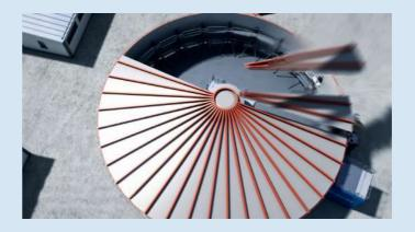
5. Assemble the roof construction - it is possible to rotate the tank with a rotating shoring tower.
