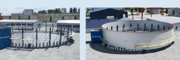
3. Place the equipment at the annular plates and assemble the Lift Jacks.
