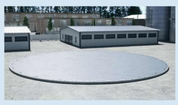
2. Place the annular and bottom plates at the foundation.
