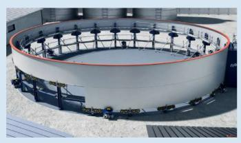
4. Feed in and tack weld the 2nd course, lower Jack one by one during the infeeding of the sheet.
